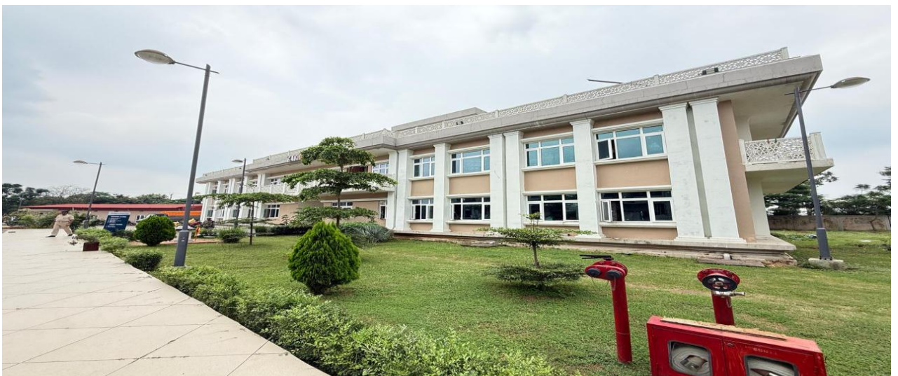
Figure 6 Site Location photograph of Existing Barrack Building
